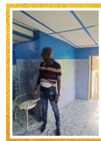
Extension of delivery room at CEM
