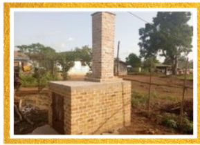
Incinerator constructed Yekepa Free Pentecostal Clinic
