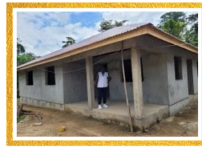
MCH construction at Doris Medical Clinic in Nimba
